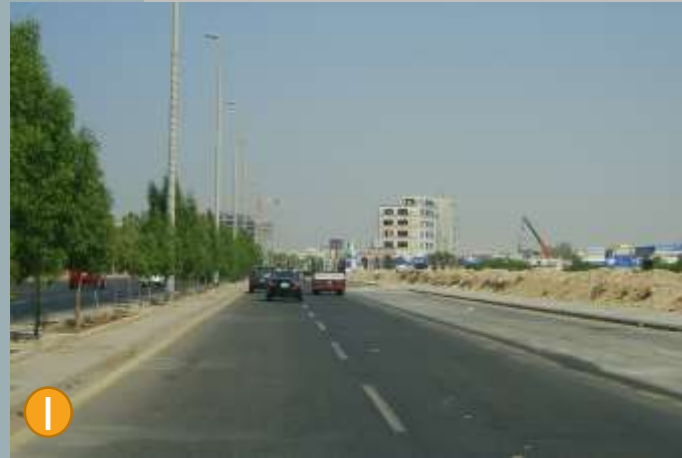
Figure 1: Al Malik Road, existing conditions
